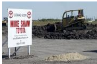
Construction begins on the new Mike Shaw Toyota dealership in Callalen.
